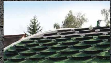
A slope interrupter system will be installed on three sides of the roof. The south-facing side has solar panels.
